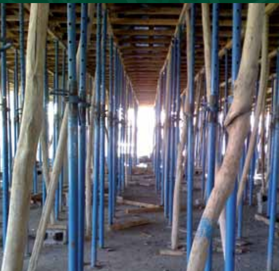
Internal shot: Structural support system used on site in Iraq.
