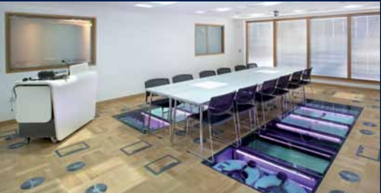
Air handling units are deliberately visible to aid teaching and learning
